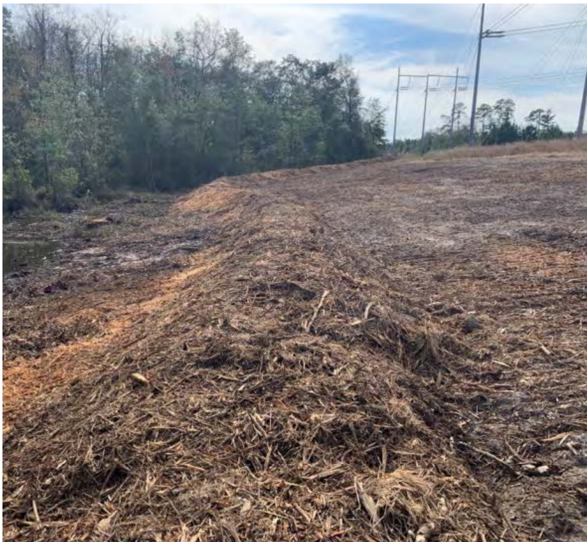
ECM berm example protecting wetland
