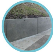
POUR-IN-PLACE RETAINING WALL
