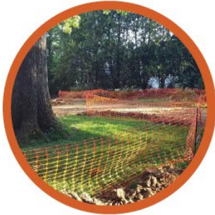
TREE PROTECTION FENCING
