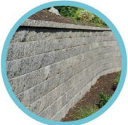
CMU RETAINING WALL
