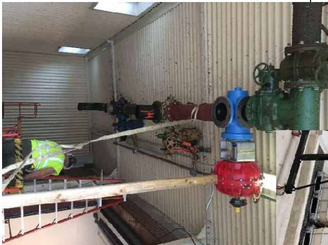
2019 CIP 416 project 3001 - Cake Unloading Valve during installation
