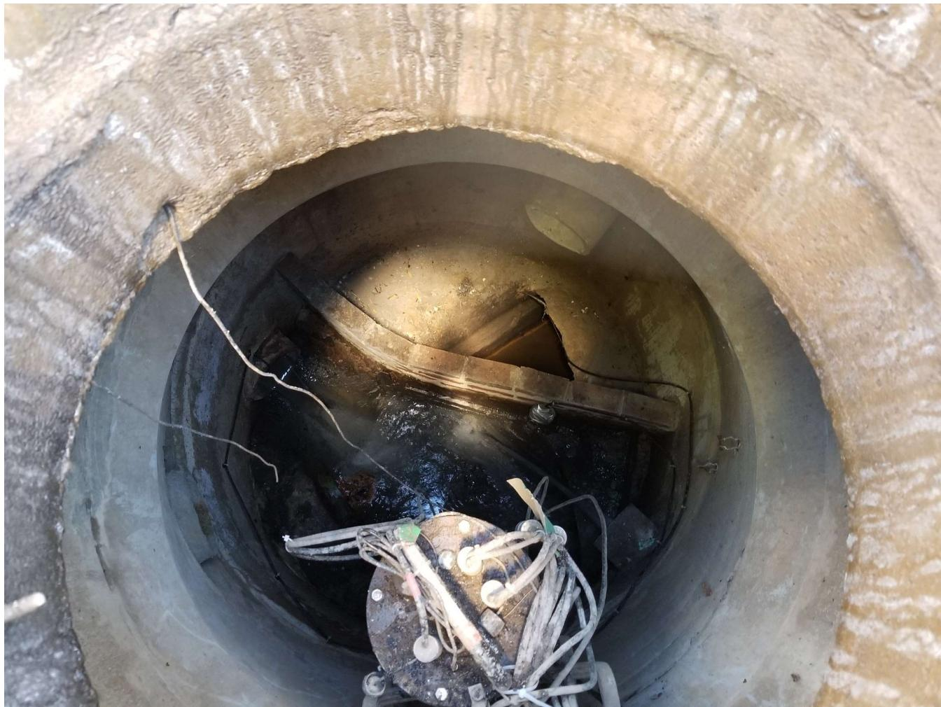
The image shows the inside of the CSO 007 regulator manhole including the CSO diversion wall in the upper half of the manhole and the monitoring equipment in the lower portion of the image.
