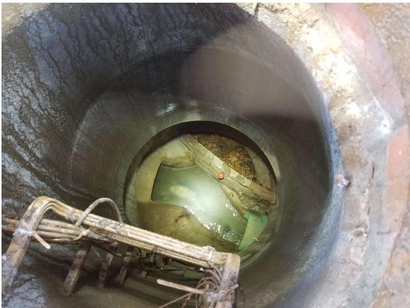
The image shows the inside of the CSO 008 regulator manhole including the CSO diversion wall in the upper half of the manhole and the monitoring equipment in the lower portion of the image.
