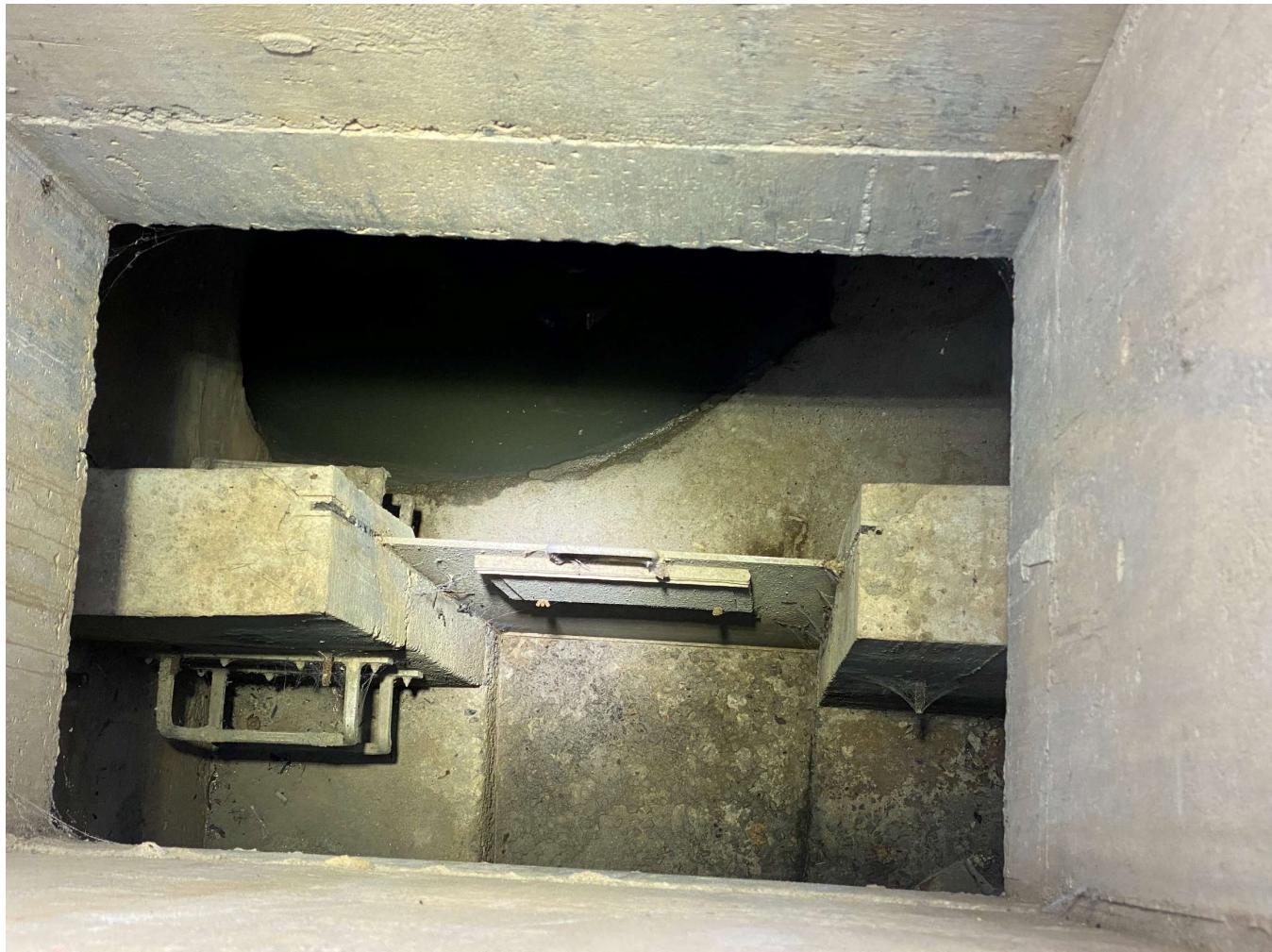
The image shows the inside of the CSO 004 regulator structure including the weir wall with adjustable weir plate. The overflow outfall channel is in the upper portion of the image.
