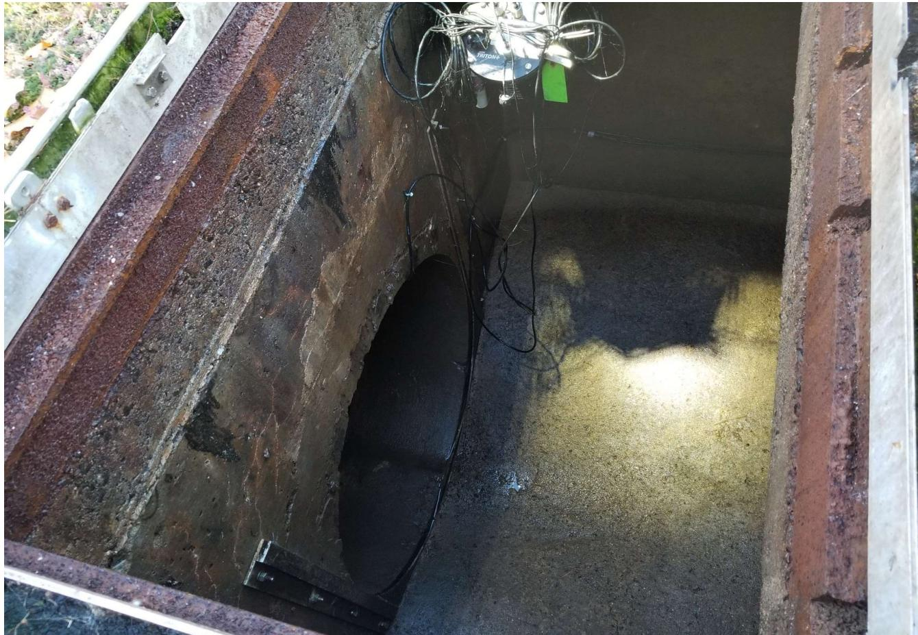
The image includes the CSO 003 overflow channel to the outfall pipe with monitoring equipment in the upper portion of the image.
