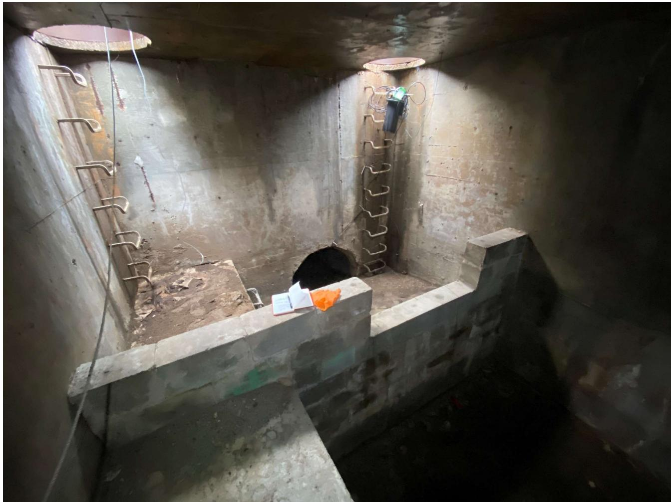
The image shows the inside of the CSO 002 regulator structure including the weir wall in the foreground of the image and monitoring equipment that is attached to the ladder rungs in the upper right-hand side of the figure. The outfall channel is in the lower right-hand corner of the image.
