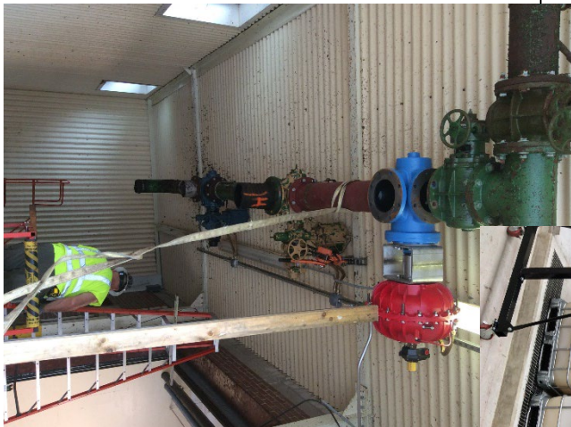
2019 CIP 416 project 3001 - Cake Unloading Valve during installation
