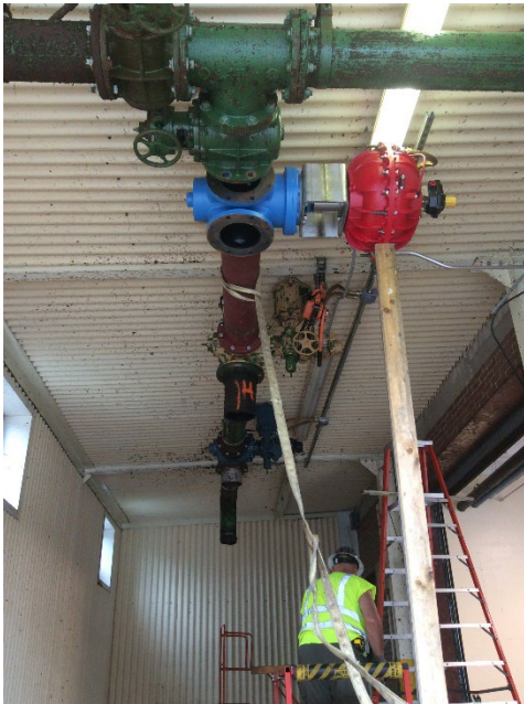
2019 CIP 416 project 3001 - Cake Unloading Valve during installation
