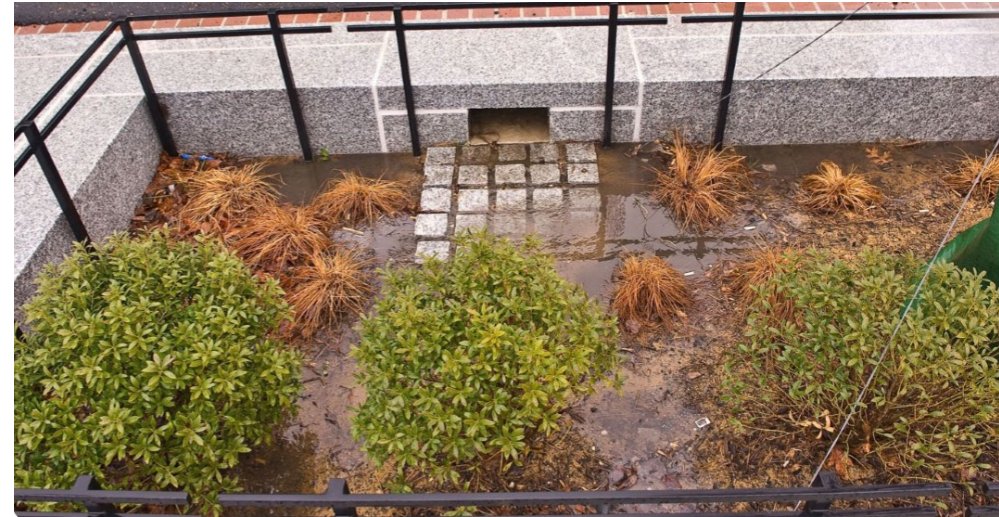
Above: Stormwater planter (bioretention). Picture credit: USEPA.
